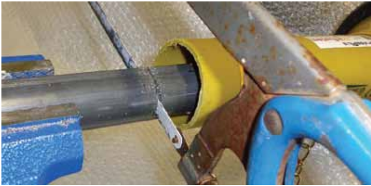
Figure 9 clamp on the part of the shaft that is being cut off then cut
